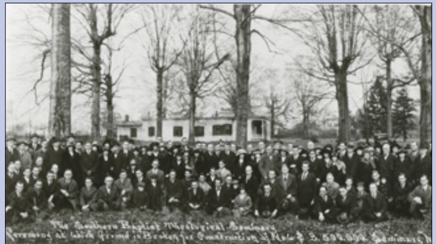
Members of the seminary community gathered for the groundbreaking of Norton Hall on the Beeches campus, Nov. 28, 1923. Photo from SBTS archives.
